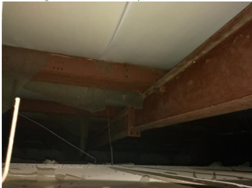
Figure 50. View of truss and purlins of Fein new church
