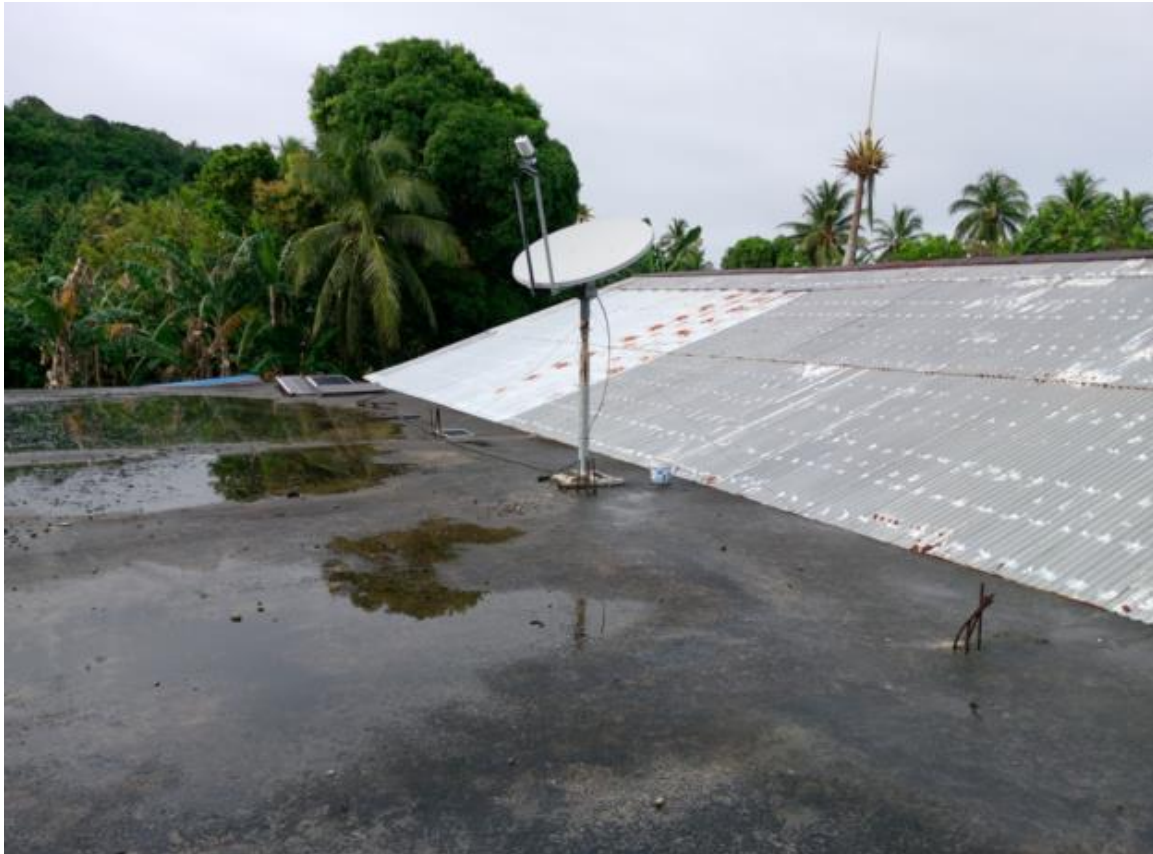
Figure 24. community building and church (right) roofs. Antenna to be removed
