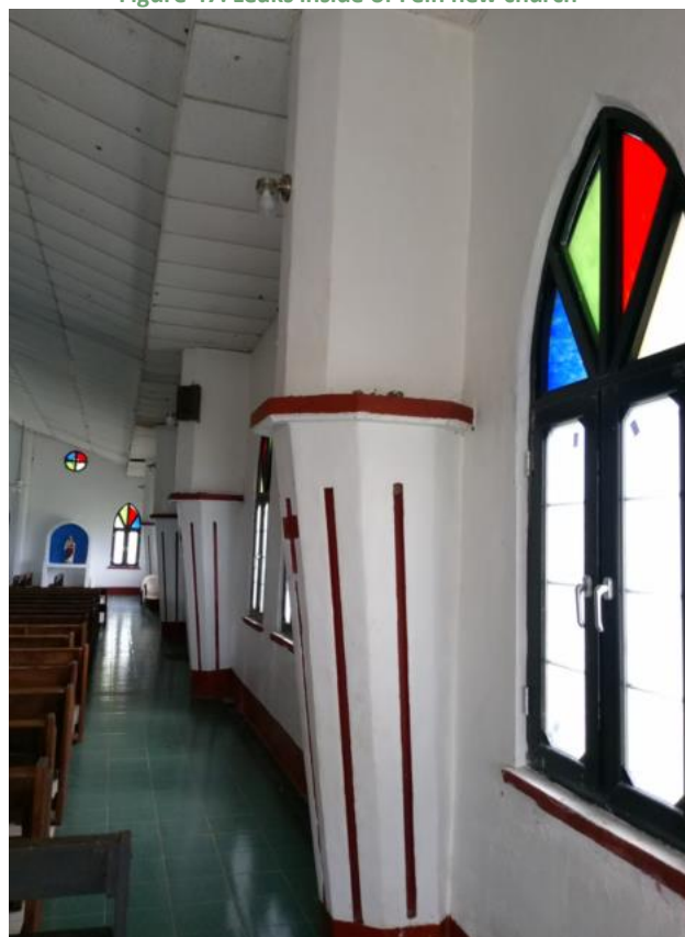
Figure 48. Concrete base of the trusses of Fein new church
