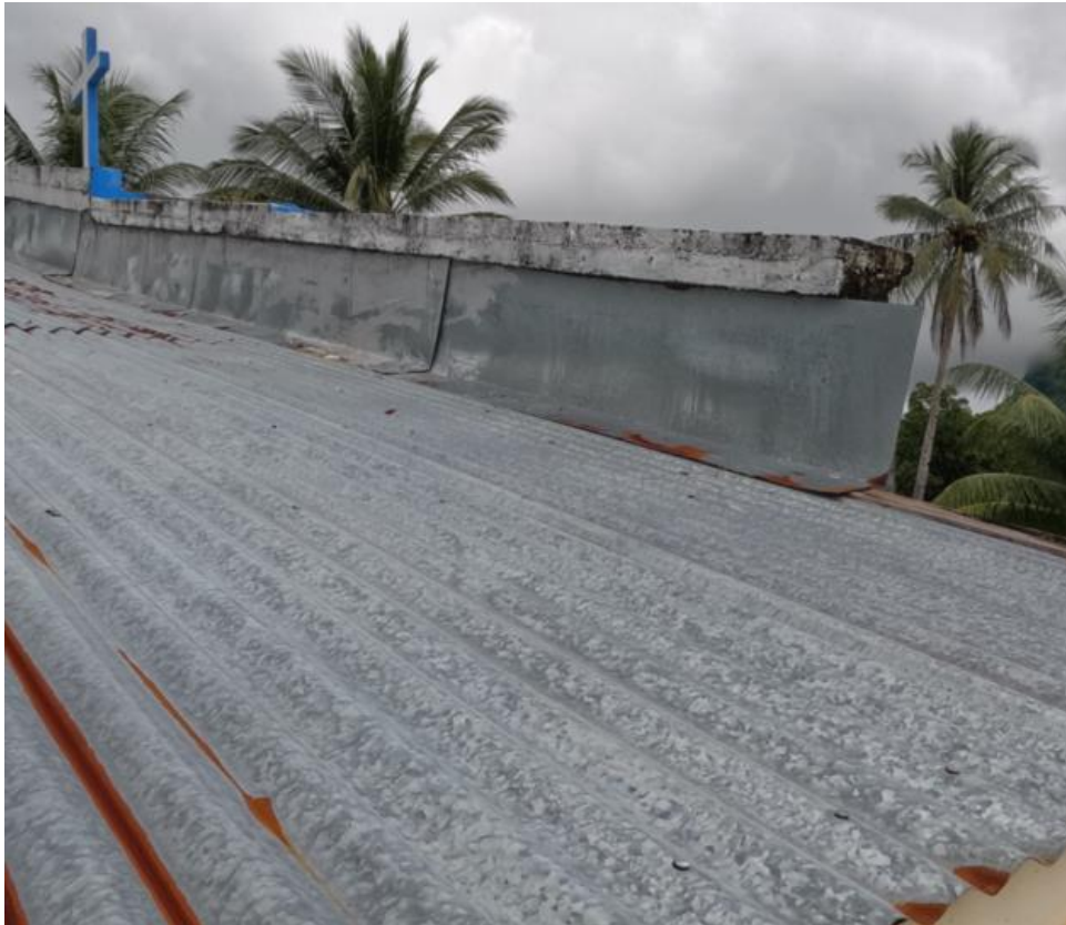
Figure 97. Mesa church roof
