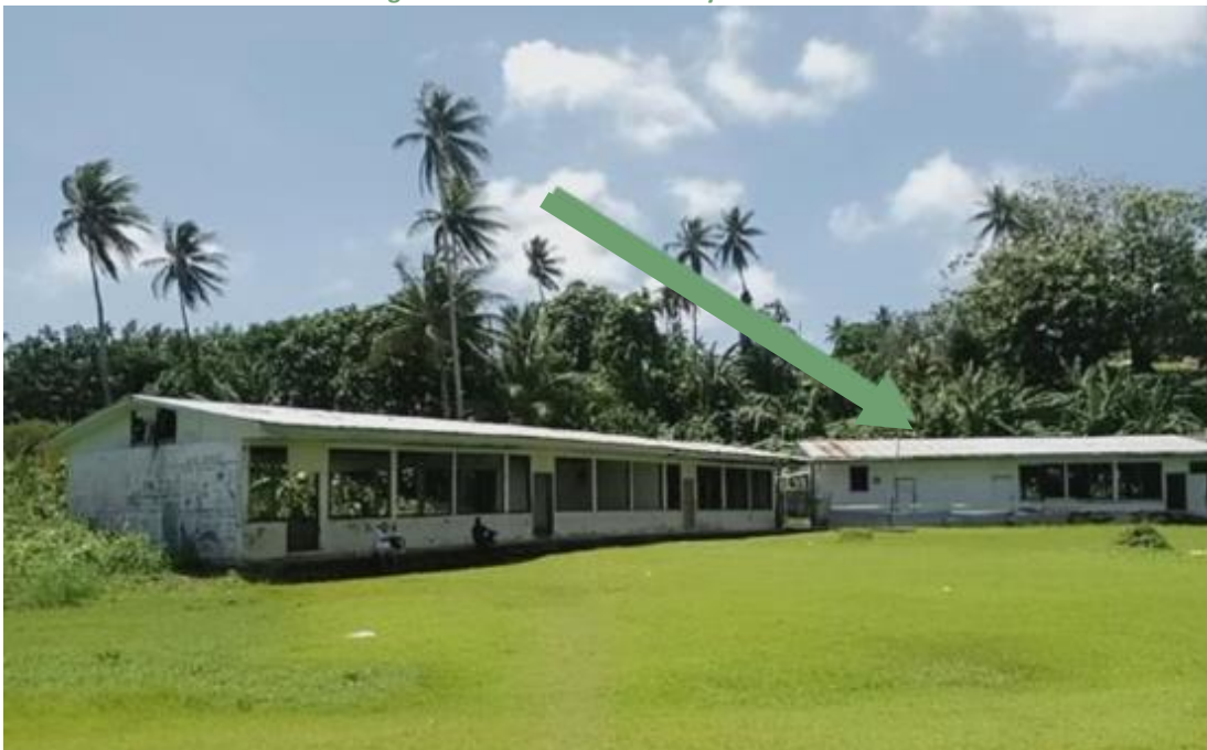
Figure 68. Distant view of roof for G3 - RT1
