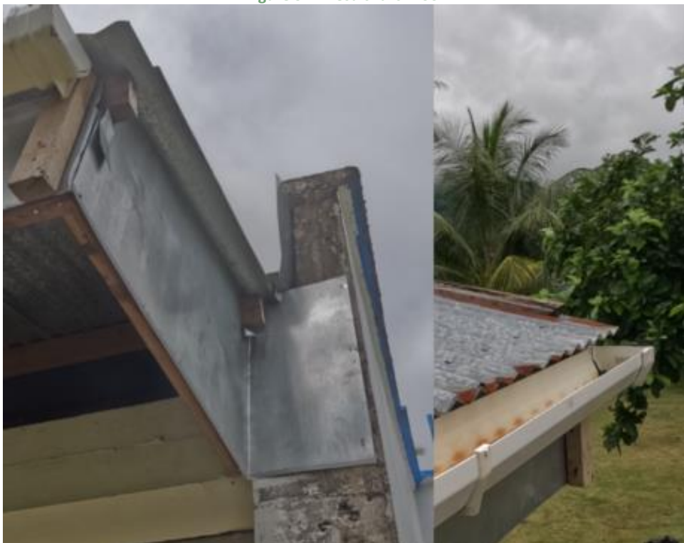
Figure 98. Mesa church roof 2 and edge (Eastern view)
