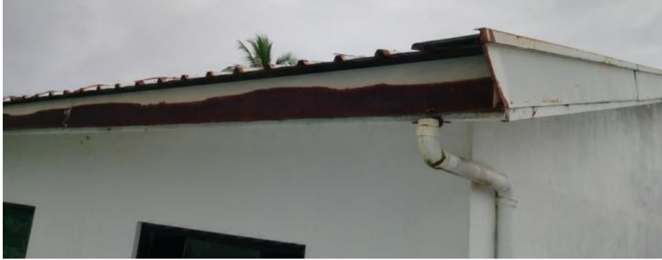
Figure 3. Edge of the Sapota 1-storey elementary school roof
