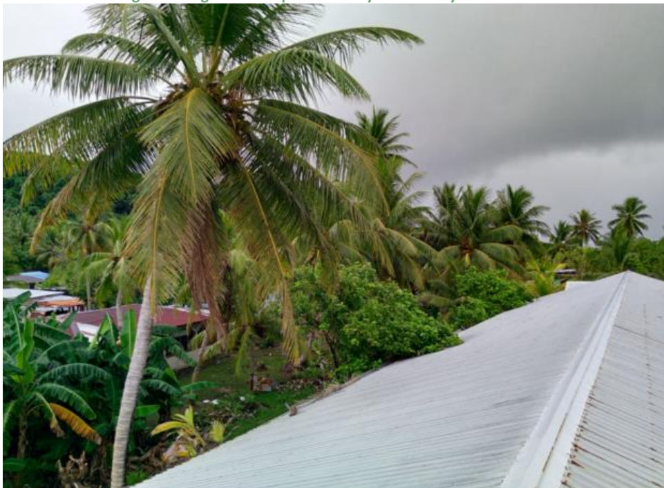
Figure 5. West part of the Sapota 1-storey elementary school roof
