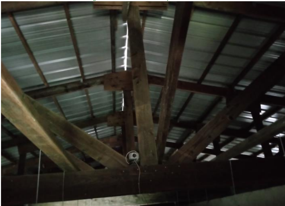
Figure 11. Roof structure of the Sapota 2-storey elementary school
