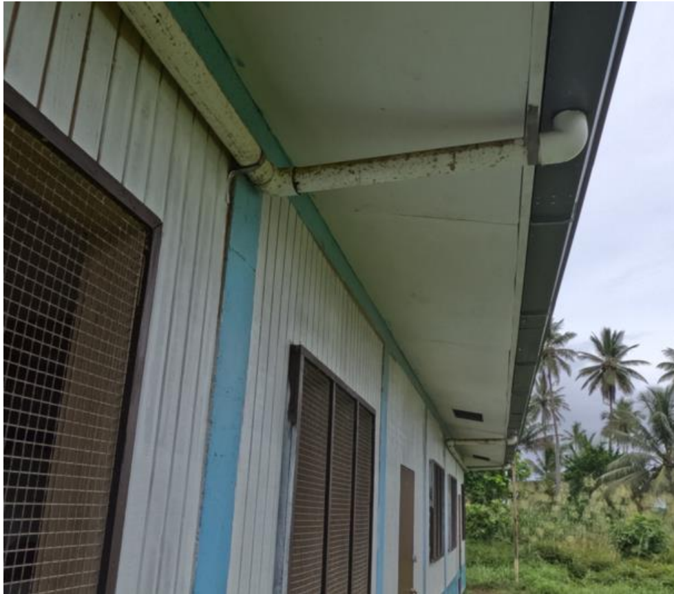
Figure 82. Side of the Mesa Municipal office displaying rain gutter
