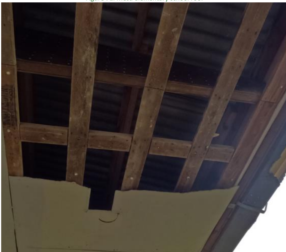
Figure 72. Wooden structure of the Mesa elementary school
