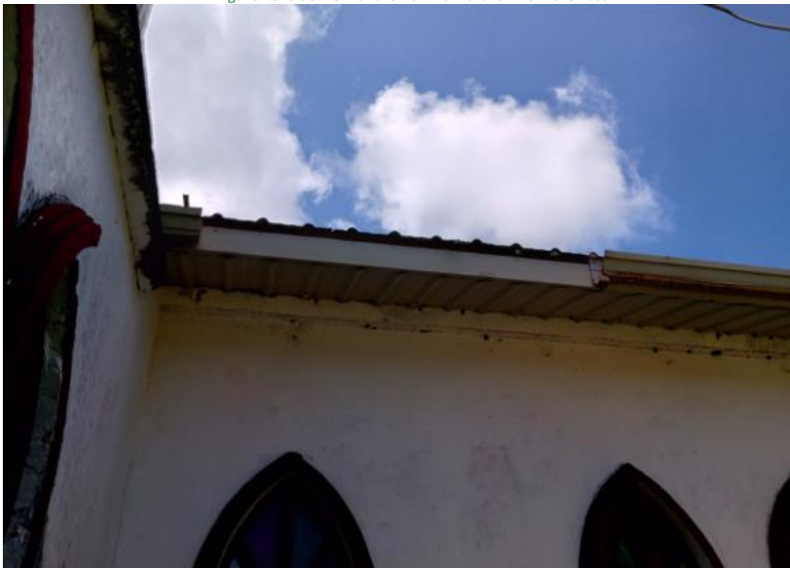
Figure 44. View of roof edge in G2-RT1
