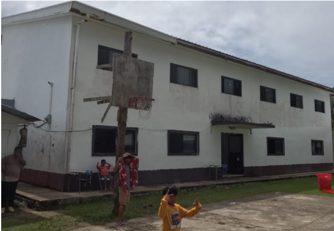
Figure 18. Sapota current warehouse (left), 2-storey high school (middle), 1-storey elementary school (right) and basketball court (bottom)
