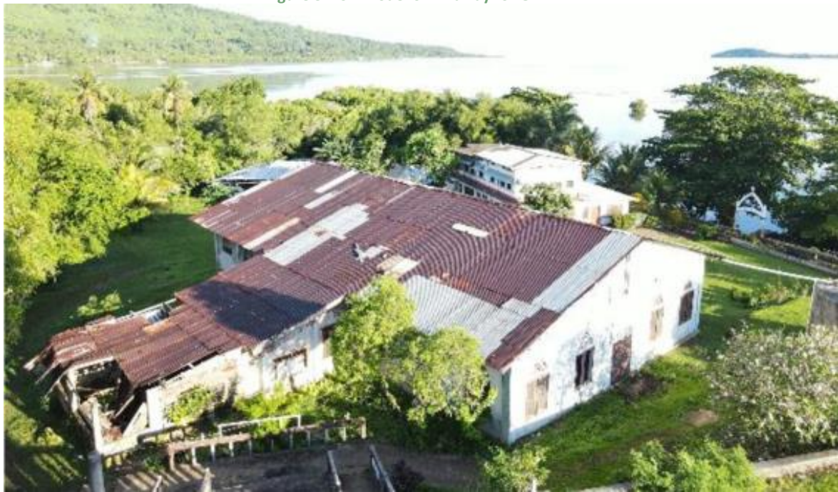
Figure 55. Aerial view of G2-RT2 roof
