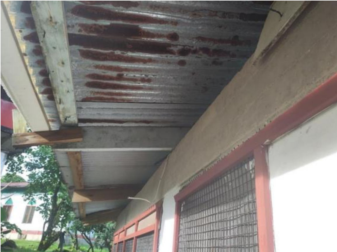
Figure 64. Parish hall roof edge
