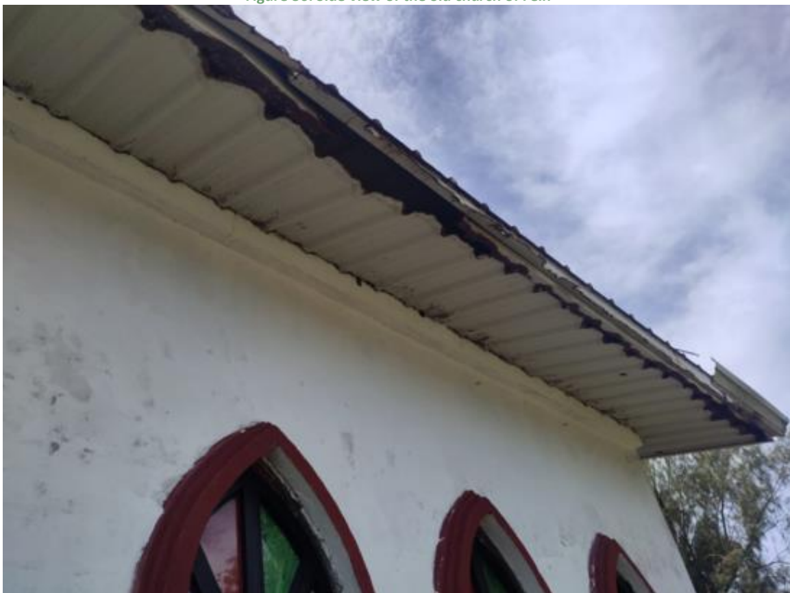
Figure 57. Roof edge of the Fein old church
