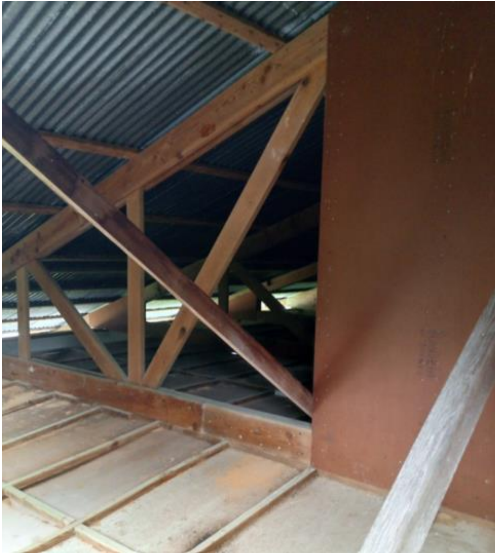
Figure 28. Sapota church roof structure
