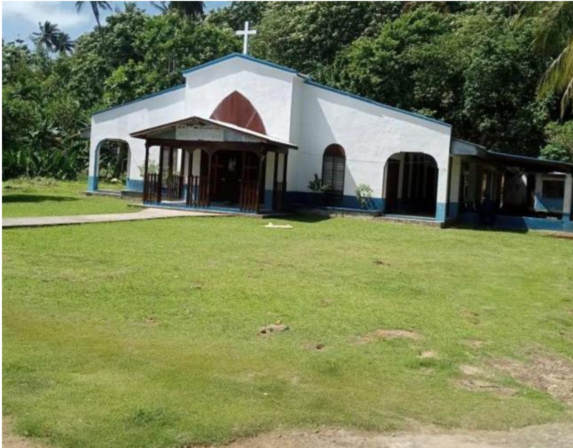
Figure 103. View of available land plot for installation of canopy
