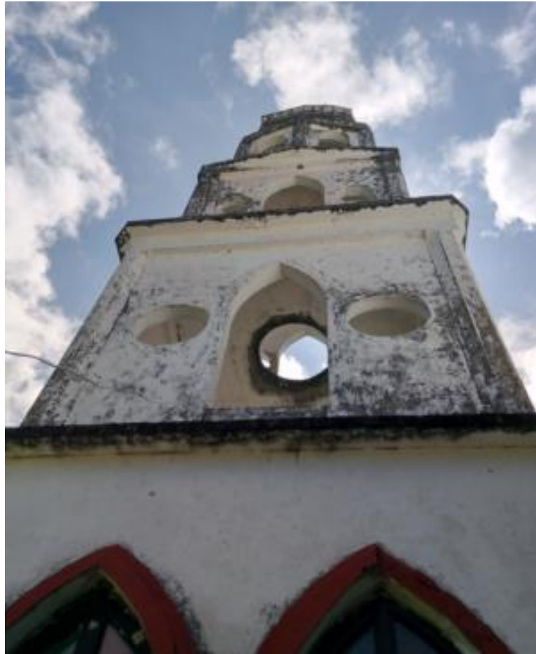
Figure 45. View of one of the two towers of Fein new church
