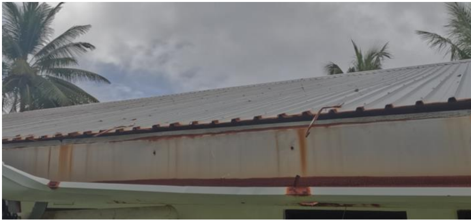
Figure 4. Edge of the Sapota 1-storey elementary school roof 2
