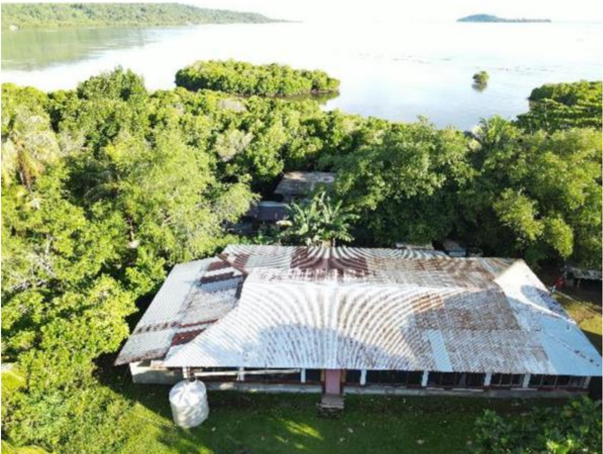
Figure 61. Drone view of roof in G2-RT3
