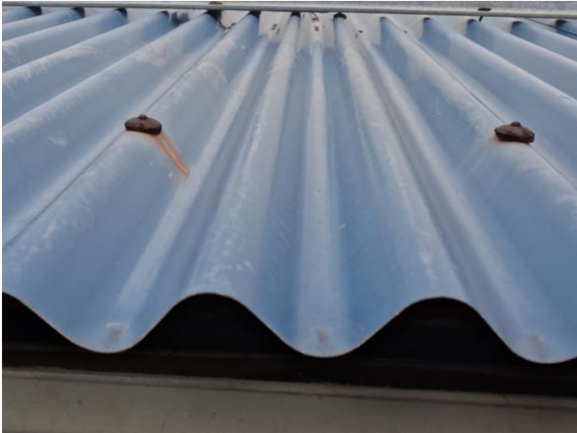
Figure 86. Edge roof of the Mesa municipal office
