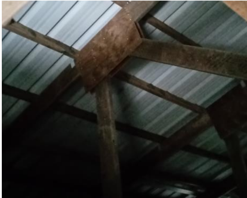
Figure 12. Figure 11. roof structure of the Sapota 2-storey elementary school 2
