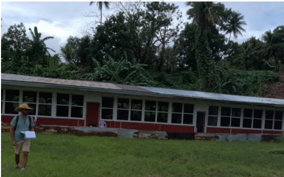
Figure 70. View of the Mesa elementary school
