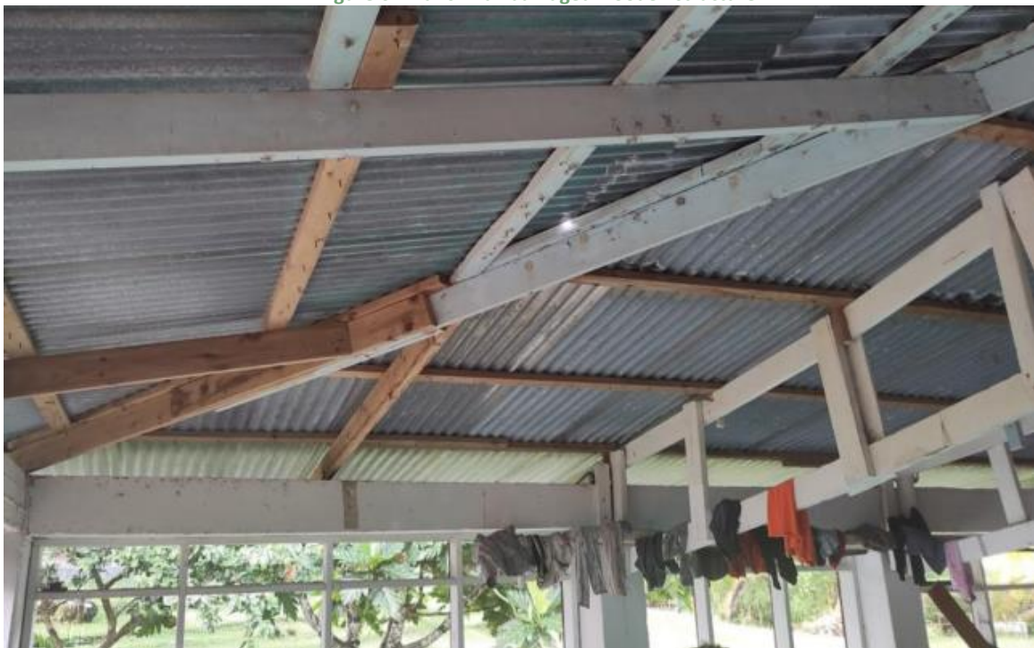
Figure 63. Parish hall wooden structure
