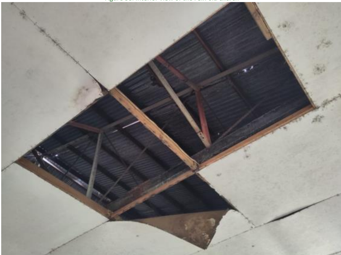
Figure 59. Steel structures of the old church's roof (truss)
