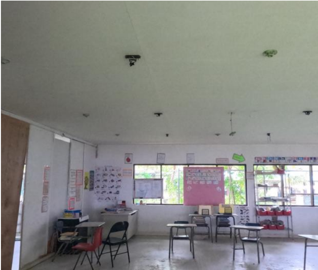
Figure 6. Sapota 1-storey elementary school interior. No visible leakage
