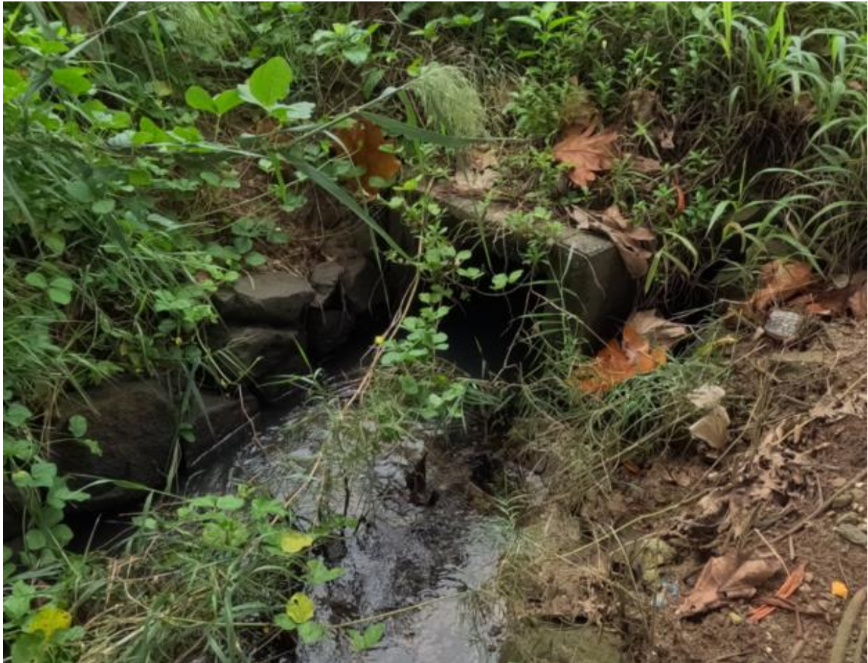
Figure 89. Small creek at Mesa, the concrete pipe is 77cm high
