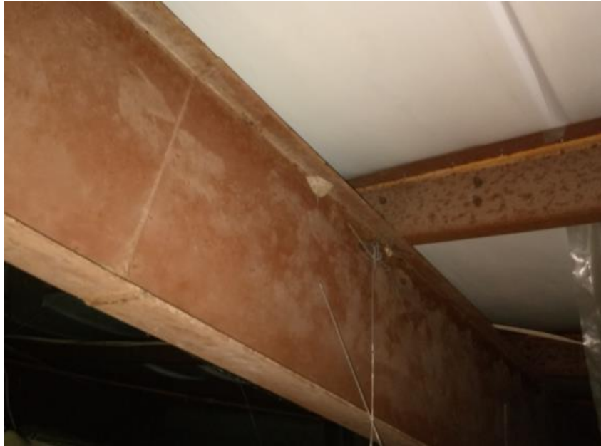
Figure 49. Junction main trusses-purlins of Fein new church
