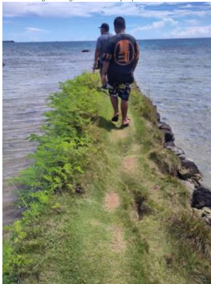
Figure 42. Jetty close to G2-RT1, approximately 100 yards to its North
