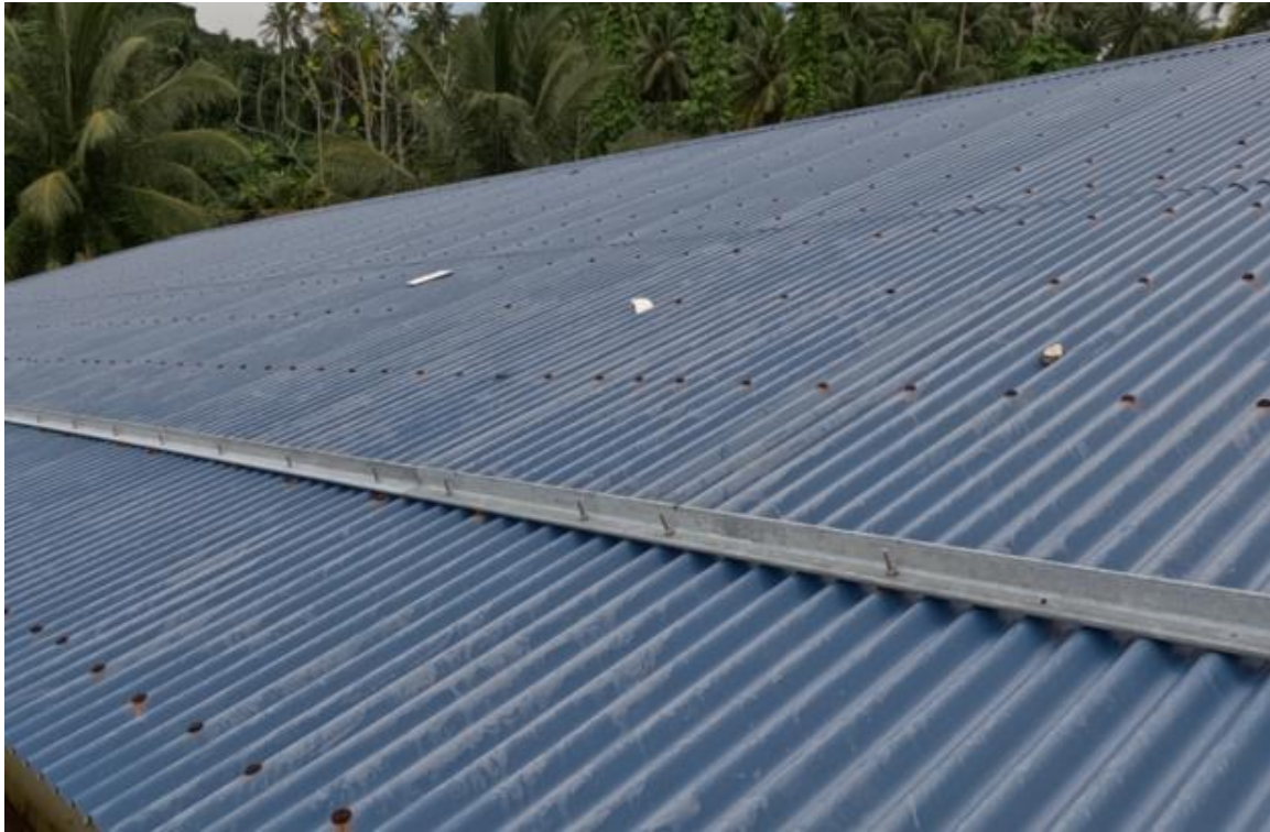
Figure 84. Roof of the Mesa municipal office
