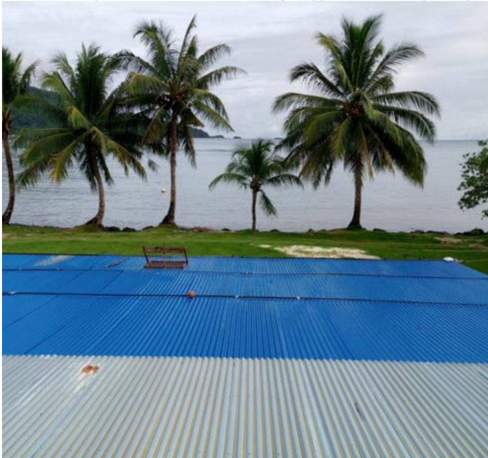
Figure 23. View of existing canopies
