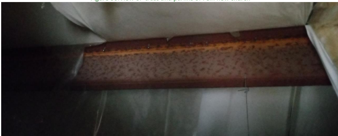
Figure 51. Steel purlins of Fein new church
