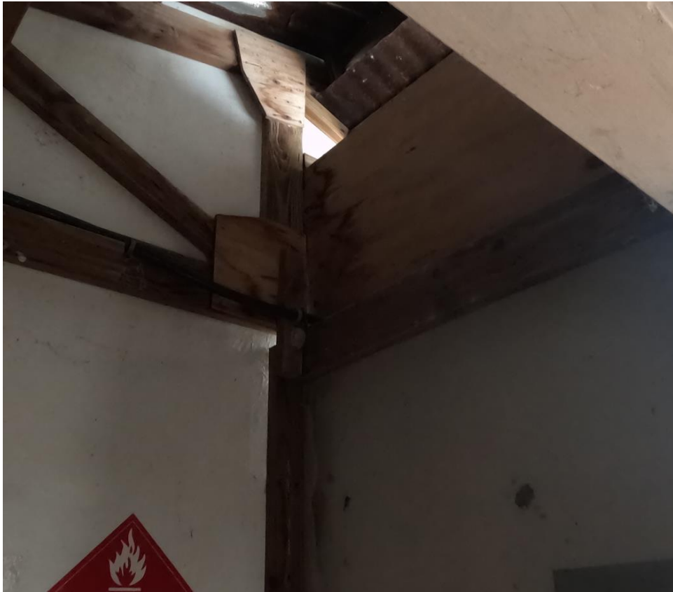
Figure 16: wall and roof structure of the technical building (current)
