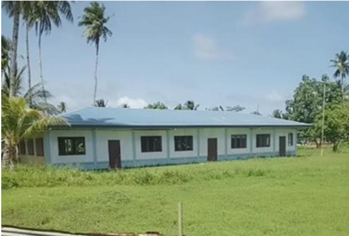
Figure 80. View of municipal office
