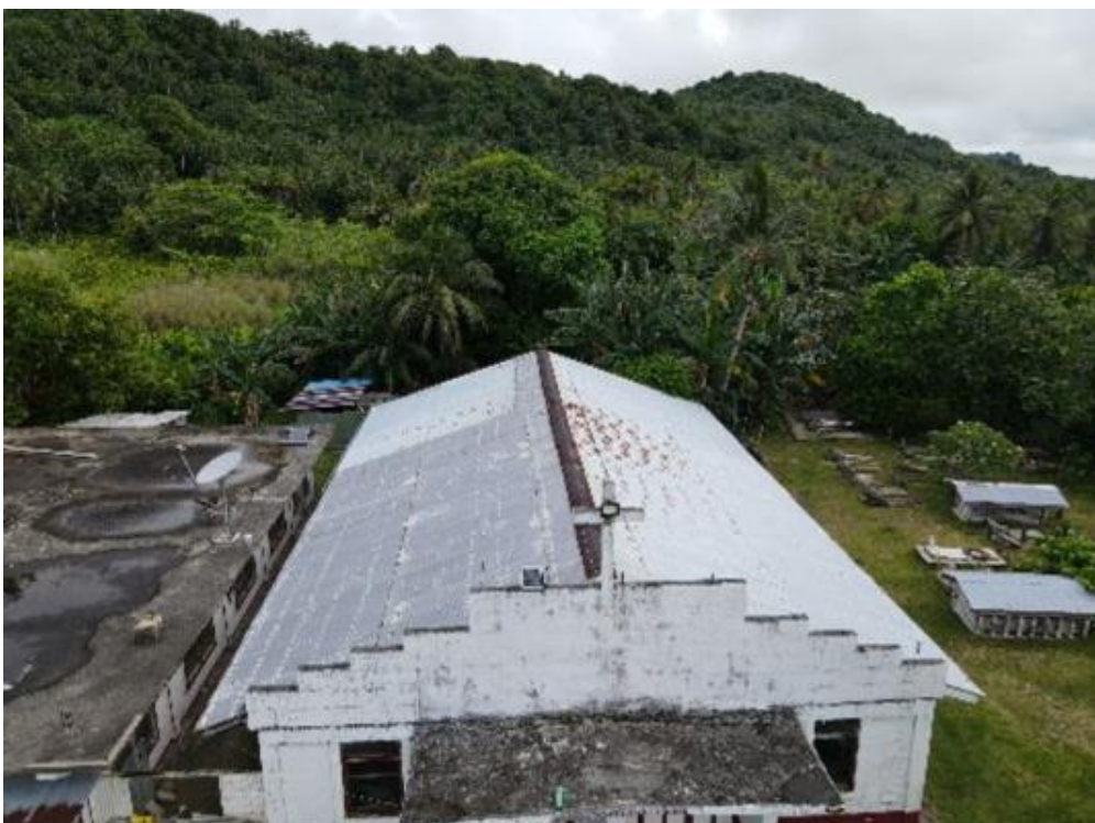
Figure 21. Drone front elevated view of roof in G1-RT3
