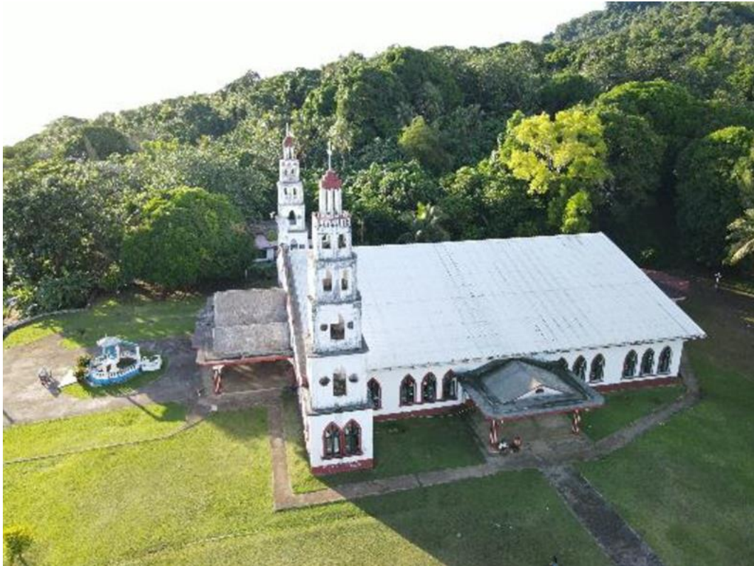
Figure 39. Drone footage of roof in G2-RT1
