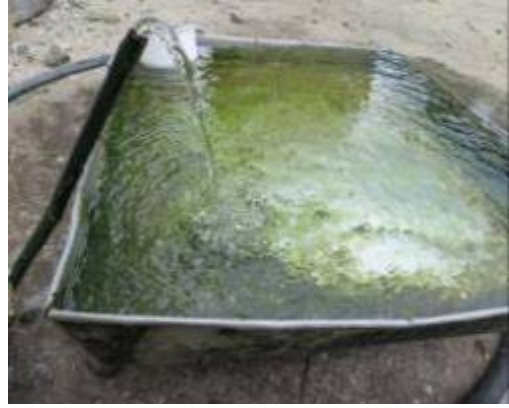
Open pipe, with continuous flow at ground level.
